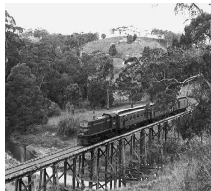
Bridge over Curdies River, c1960
